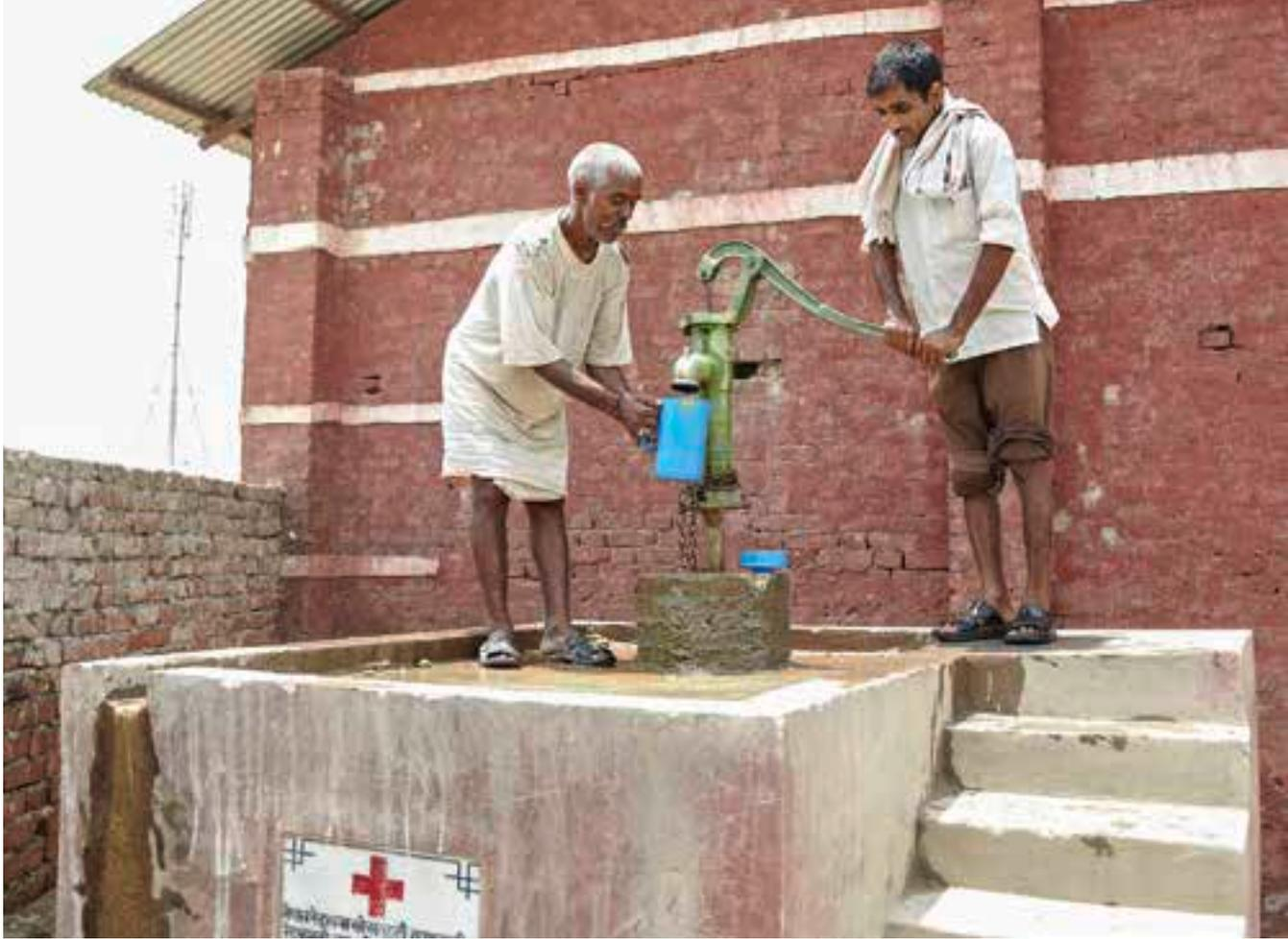
The raised water point provides clean drinking water even in times of flooding.
